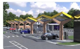
Electric Vehicle charging
